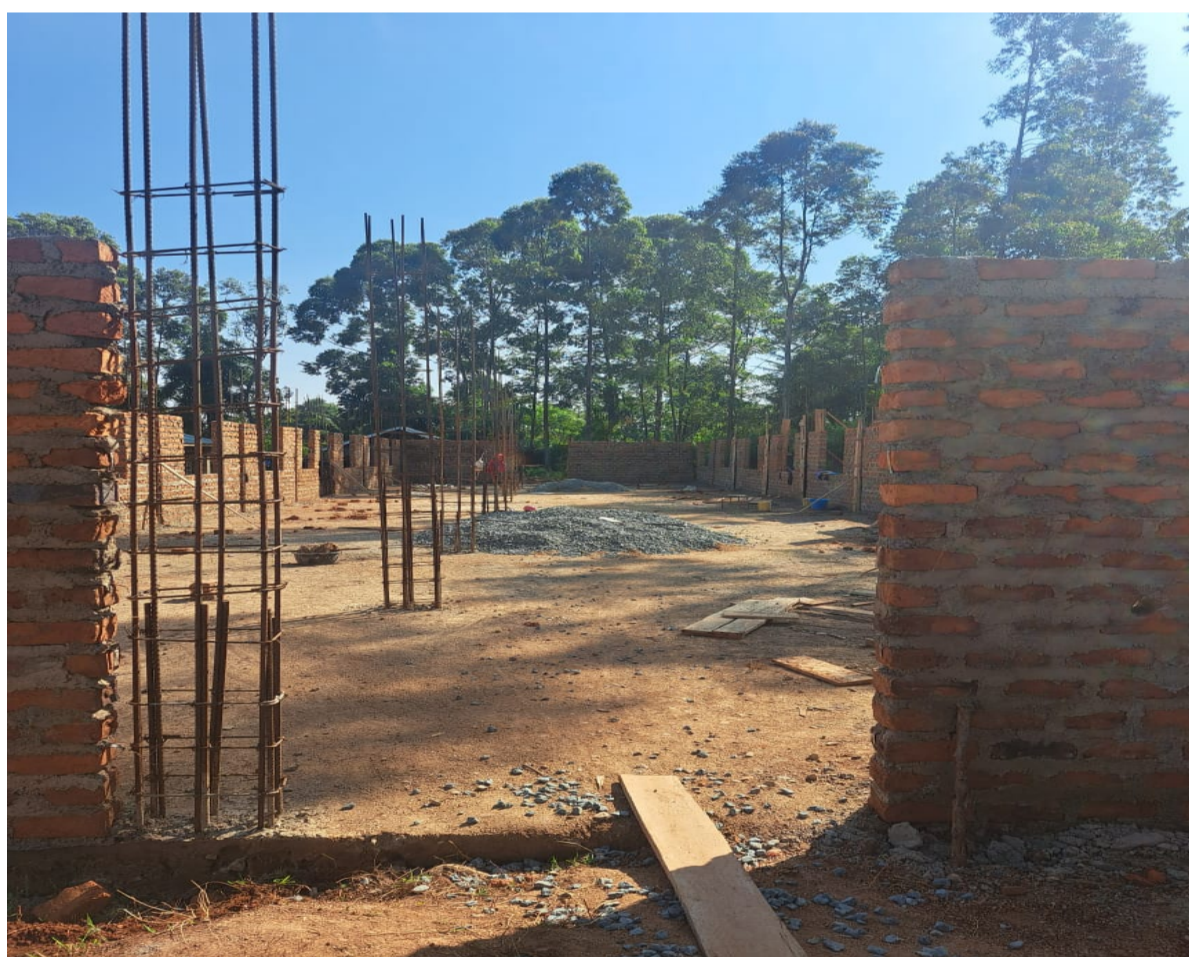
————— A dormitory under construction to accommodate the growing number of Students —————
